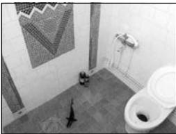
A dry urine-diverting toilet installed in a residential building in Stockholm.
